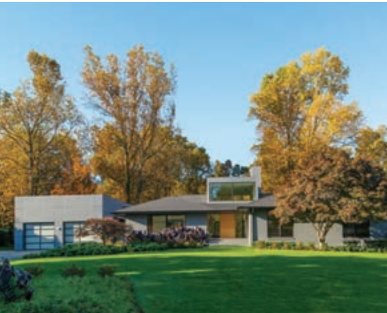
Gurney updated the exterior (above) by painting the existing bricks in gray and sheathing the garage in fiber-cement panels. In the kitchen and breakfast room (right), the orange light fixture by David Weeks Studio and chairs by KFF punctuate an otherwise neutral palette of marble countertops, wenge floors and rift-sawn, white-oak cabinetry.
