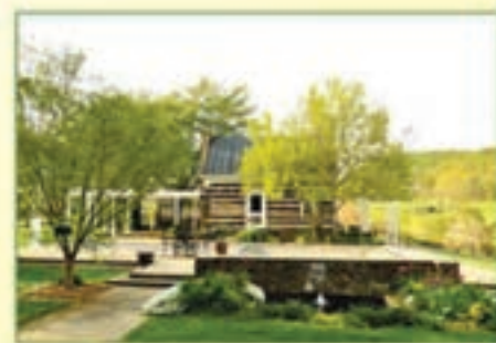
Guest House ~ Pool House
