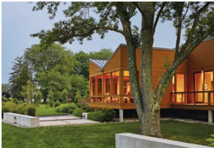
JURORS' CITATION Treacy & Eagleburger Architects PC, Grays Inn Creek House, Rock Hall, Maryland. Photography: Alan Karchmer.
