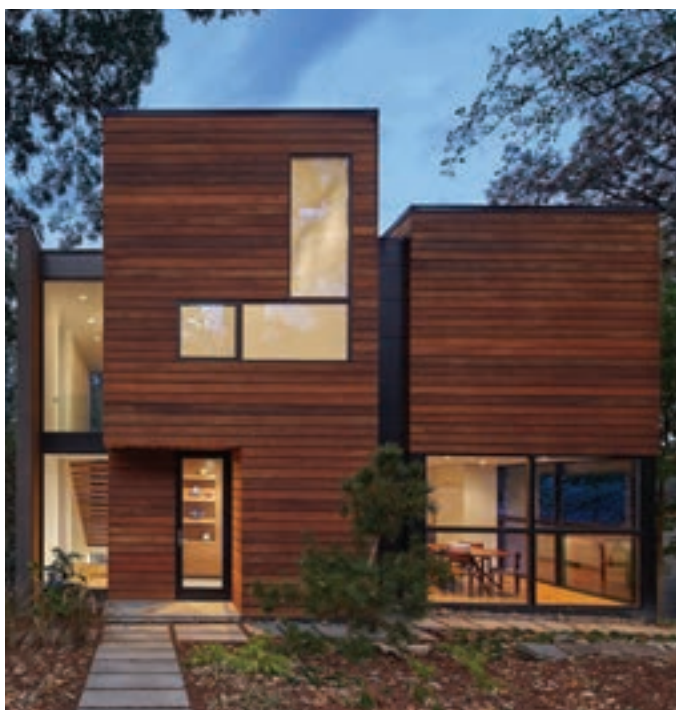
AWARD OF MERIT Robert M. Gurney, FAIA, Architect, Lyon Park House, Arlington, Virginia. Photography: Anice Hoachlander.
