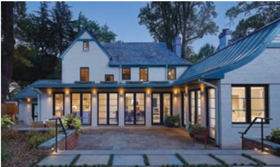
Thorsen Construction renovated a Northwest DC home in classic style. © Anice Hoachlander.
