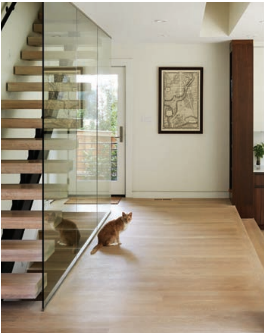
The new stairway (above) leads to the second-floor bedrooms, where the hallway is designed like a bridge flanked by open slots that let daylight filter down to the heart of the house. A panel of glass next to the stairs (inset) ensures safety while allowing for light.
