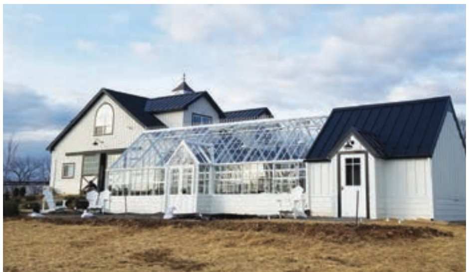
Alexander Design/Build Group—Grand Award for Residential Detached Structure. PHOTO: SOSHELUILDER
