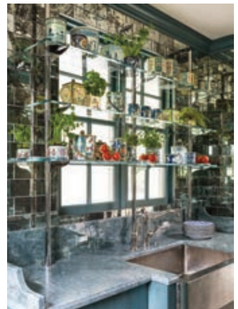
TOUCH OF GLAM Shazalynn Cavin-Winfrey of SCW Interiors tapped AK Metal Fabricators, Inc., to create a shelf system in a glamorous scullery she was designing for clients in Alexandria. A stainless-steel frame in a mirror finish supports tempered-glass shelves; the system complements a backsplash of antiqued-mirror panels. akmetalfab.com PHOTO: ANGIE SECKINGER
