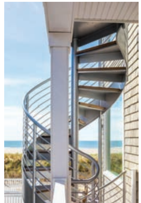
SEASIDE STYLE Pennsylvania-based Compass Ironworks was hired to design, fabricate and install a third-floor exterior stair on a Jersey Shore condo. The result was a sleek, high-grade aluminum spiral stair, powder-coated in an eco-friendly finish to withstand the harsh oceanfront environment. compassironworks.com PHOTO: DONNA CHIARELLI
